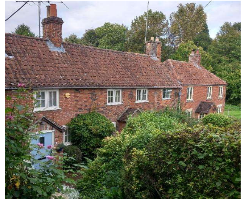
Photo 15 - Terraced cottages in Stradbrook character area
