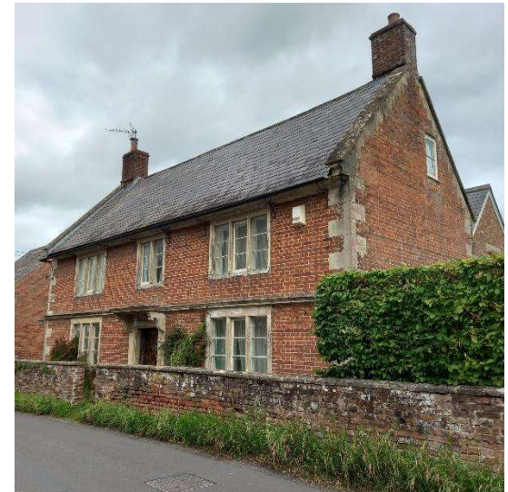
Photo 13 - c.1700 house in Braectun
