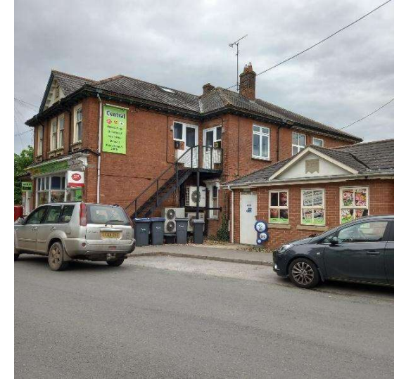
Photo 10 - Bratton Village General Stores & Post Office
